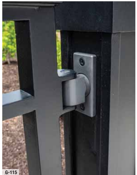
Gate hinge detail
