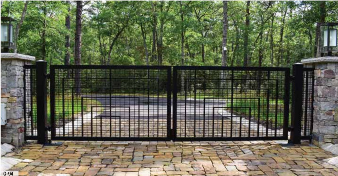
Modern Driveway to meet 4" pool code requirements.
