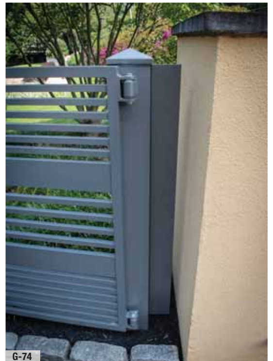
Hinge post installed behind masonry column.
