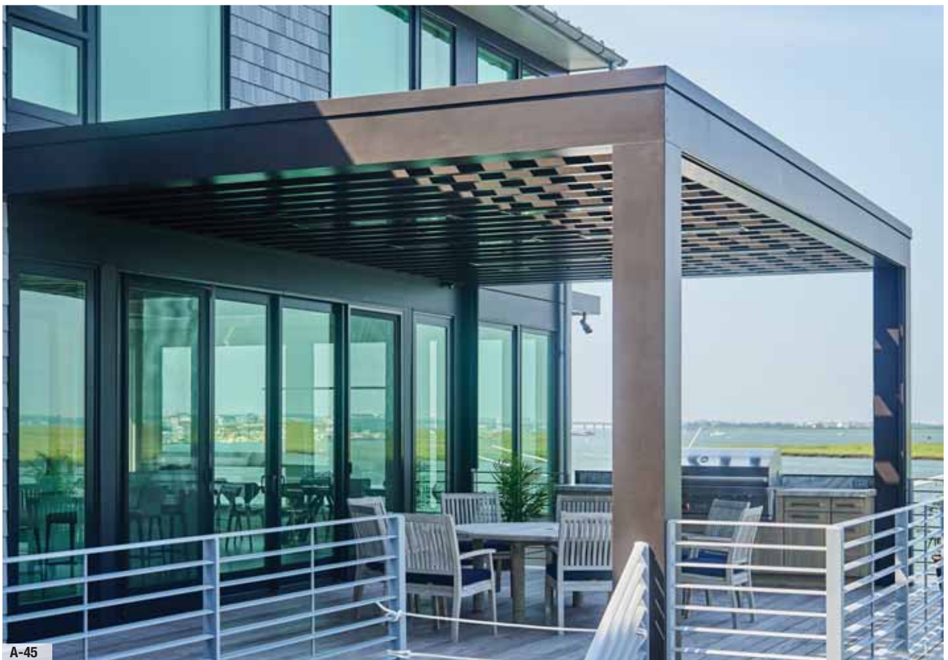
A-45 Pergola that incorporated lighting, sound system, heat, and side shade screens for a year round comfortable entertainment area.
