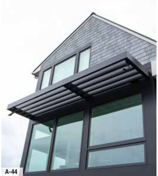
A-44 Side mounted pergola to provide shade to the inside of the home.
