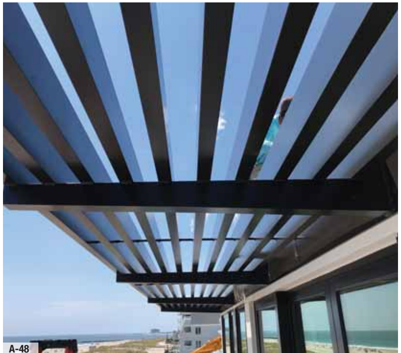
Pergola cantilever system off exterior wall.
